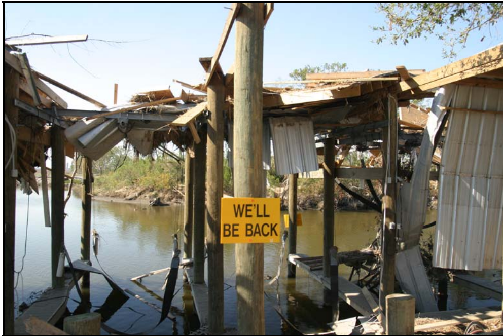
Figure 34: Marina in Lafourche Parish. Source: IAI Staff, October 2005.
