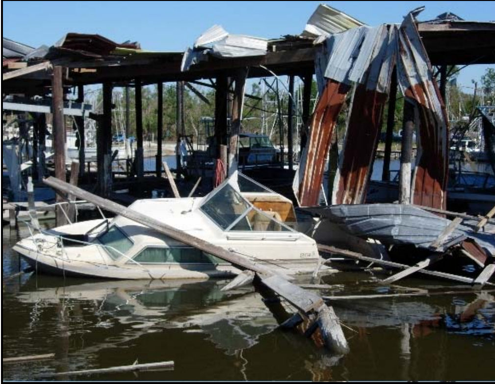
Figure 21: Lafitte (Jefferson Parish) in the Wake of Wind Damage from Hurricane Katrina and Surge Damage by Hurricane Rita. Source: IAI Staff, September 2005.
