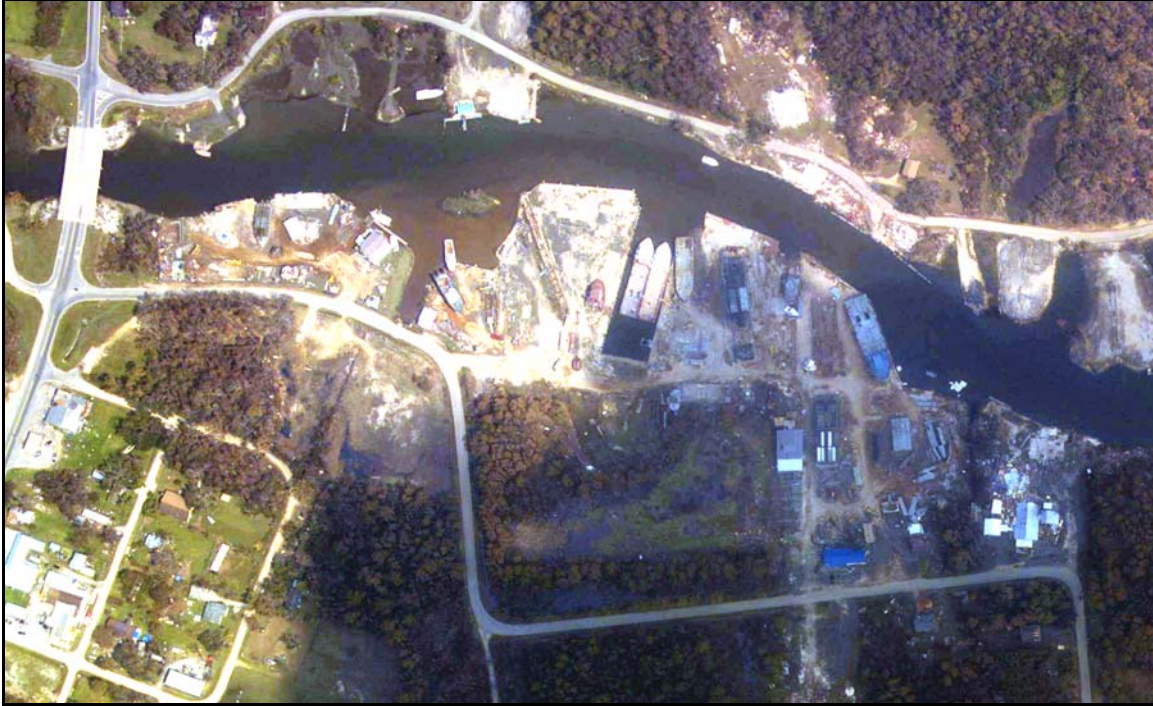
Figure 93. Bayou Coden, Entrance to the Bayou, Post-storm Surge (aerial). Source: NOAA, September 2005.
