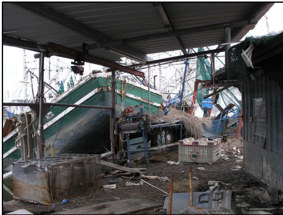
Figure 50. Offloading Dock in St. Bernard Parish with Grounded Vessels Blocking Operations.
