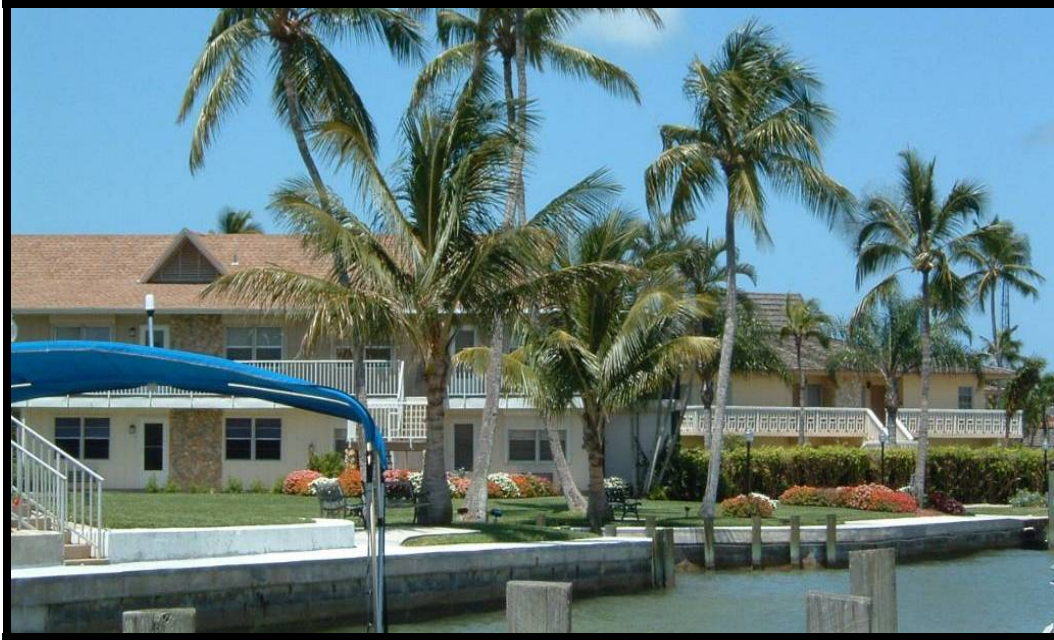
Condominiums on Marco Island
