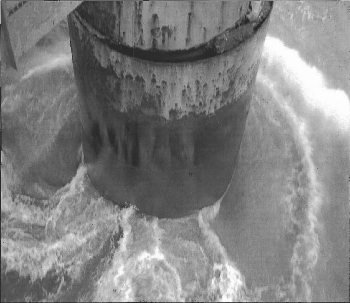
Figure 4-3 Tidal Flow around Platform Leg at Shell Platform A, Autumn 2003
