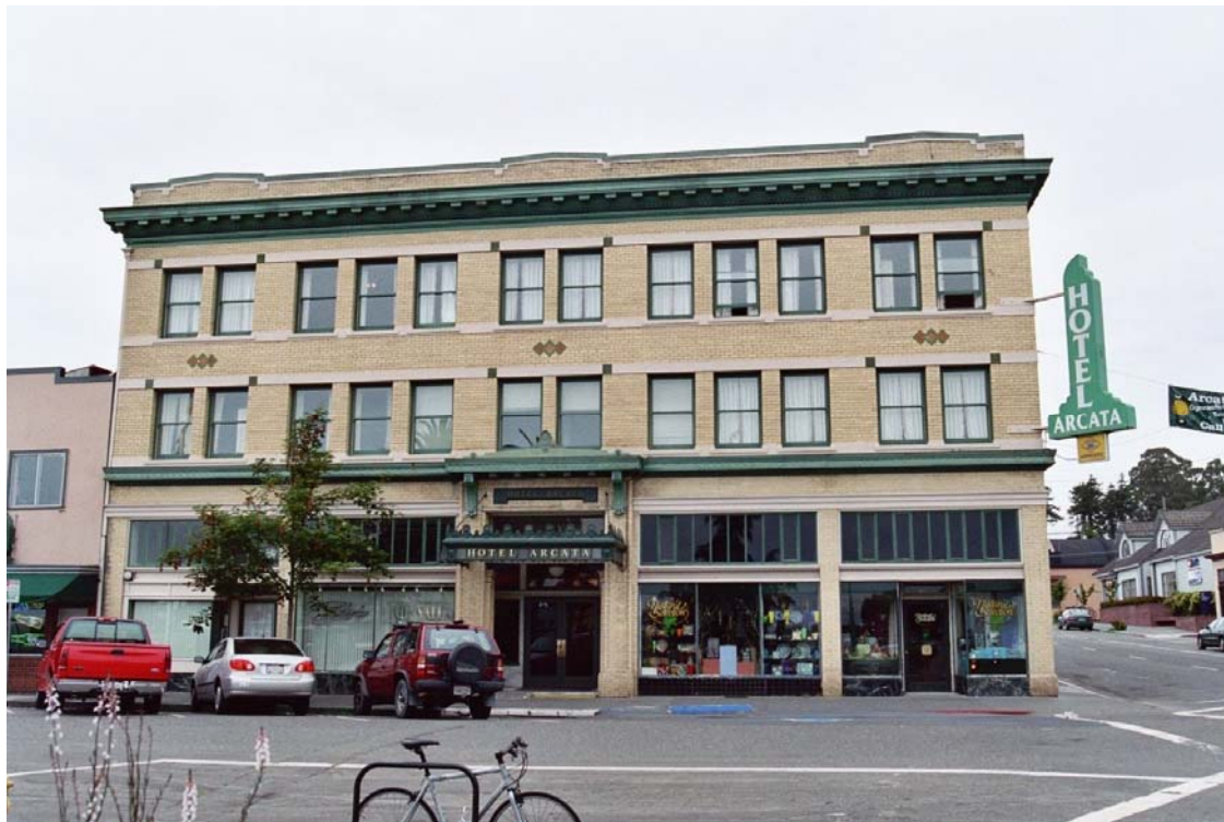
Big Lagoon Tribal Office: Hotel Arcata
