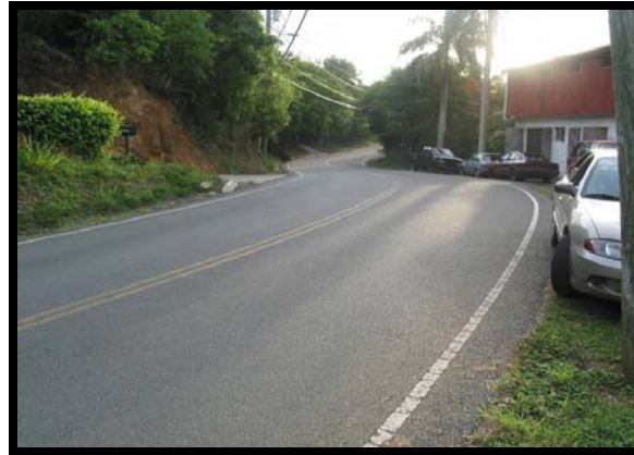
Narrow Highway 33 above Caret Bay
