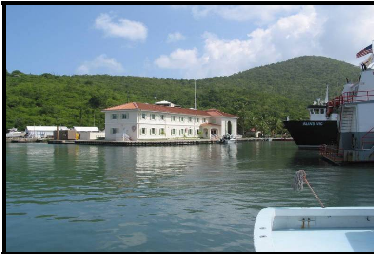
Coast Guard Building at Cruz Bay Harbor
