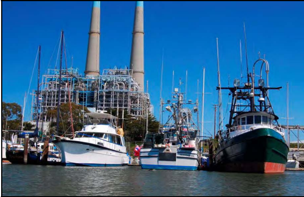
Moss Landing Harbor with Utility Plant in Background
