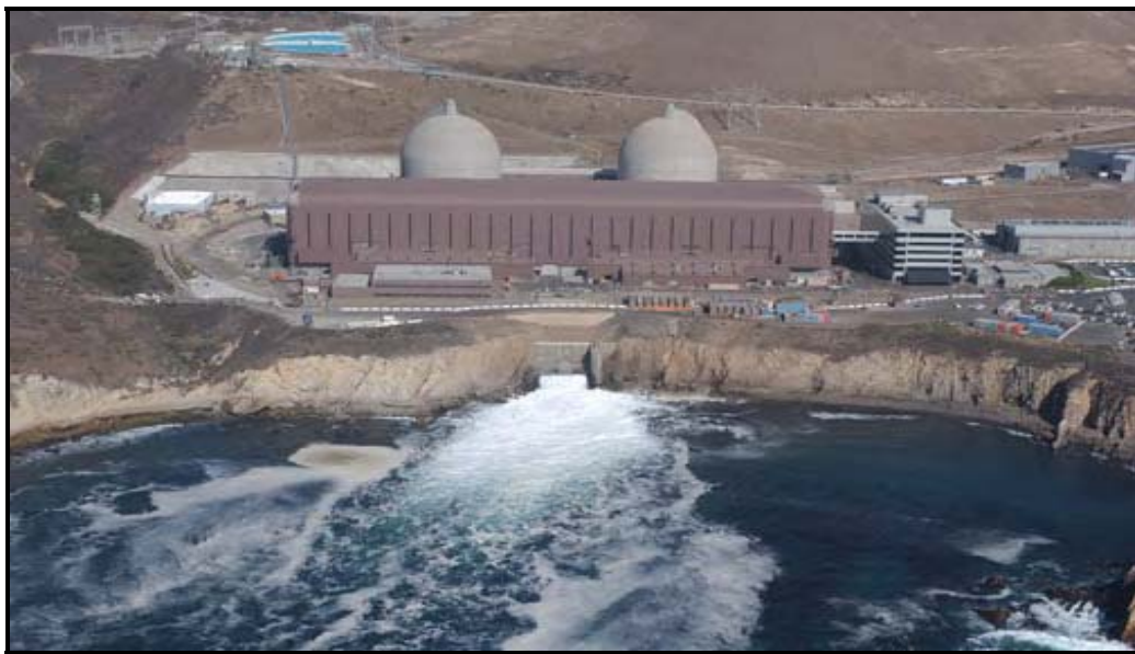
Diablo Canyon Nuclear Power Plant between Avila Beach and Montaña de Oro State Park ( www.Californiacoastline.org )
