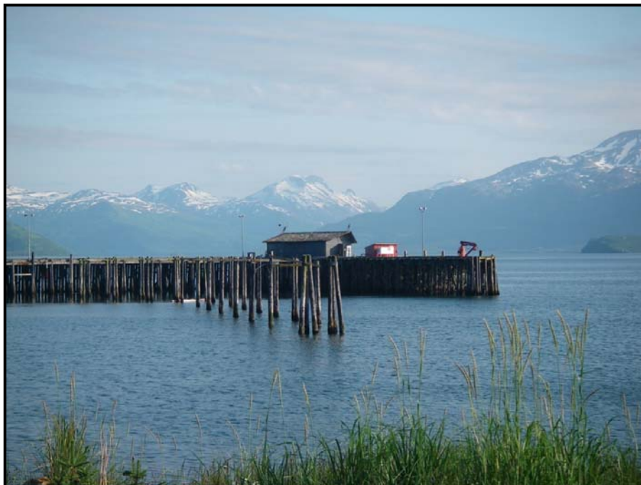
Figure 6-12 Ferry Pier at Port Lions, 2009
