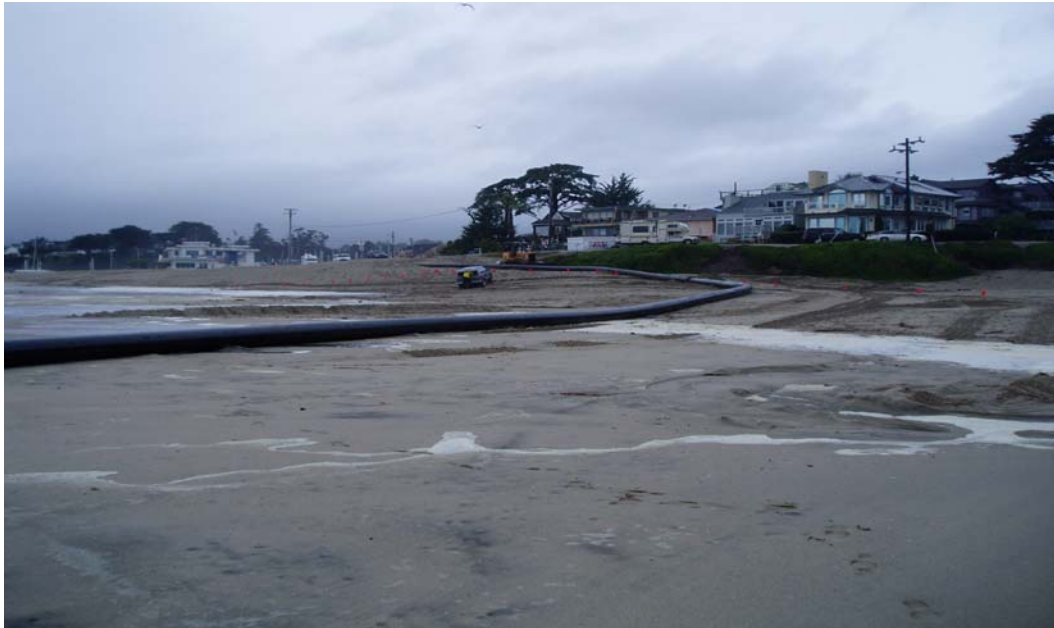
Photo 3. Disposal Onshore with Air Monitoring Occurring in the Vehicle with the Nearest Neighbors in the Background, Santa Cruz Harbor, Santa Cruz County, California
