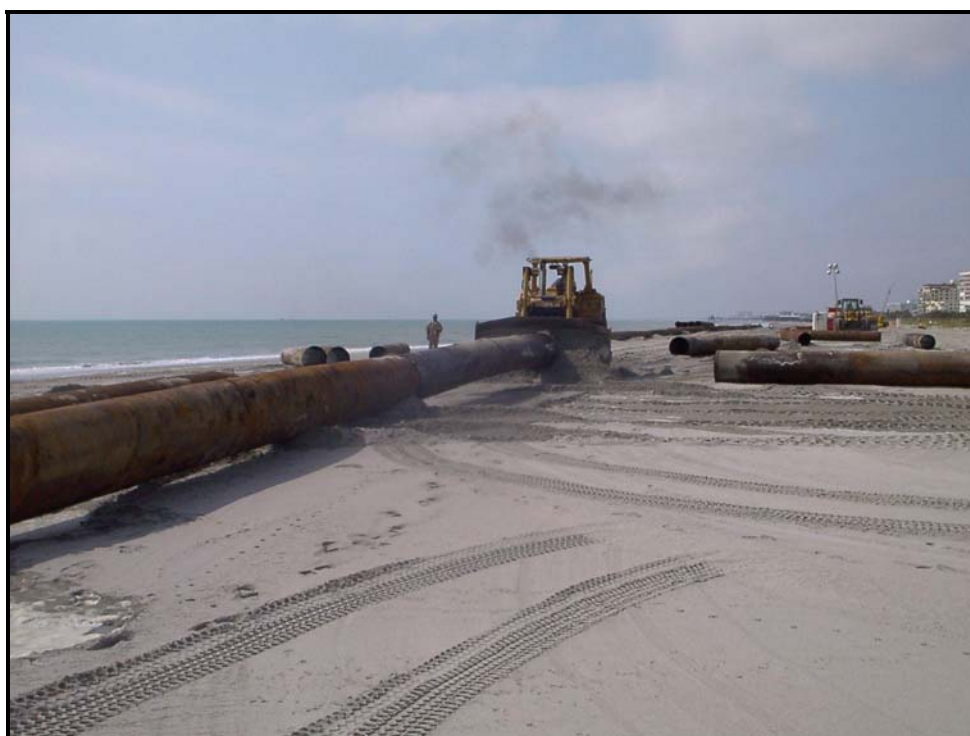
Figure 7. Pipeline along the Cocoa Beach Shoreline (IAI, 2005).
